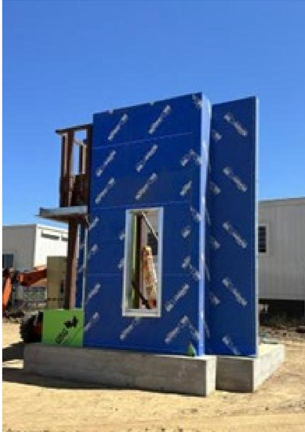
The mock-up construction started, with prefabricated metal panels installed. The Mortenson Team and Trades are forecasted to move into “Trailer City” August 16<sup>th</sup>.
