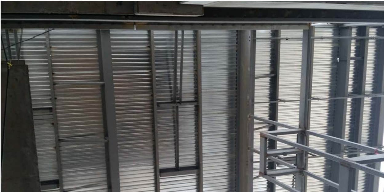
Third Floor Lobby Rough Structural Roof Framing
