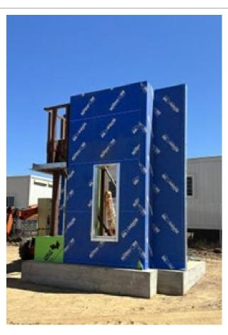
The mock-up construction started, with prefabricated metal panels installed. The Mortenson Team and Trades are forecasted to move into "Trailer City" August 16<sup>th</sup>.
